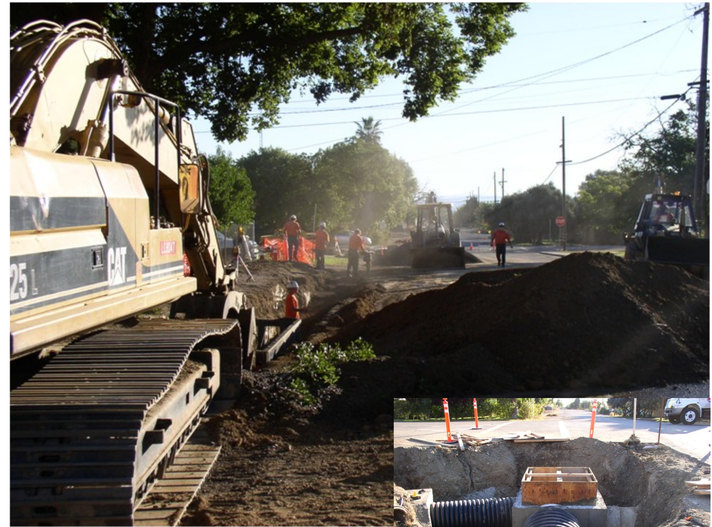
Above: Trenching on Fourth & Main in Hamilton City. At Right: Drain Inlet, also on Fourth & Main.
